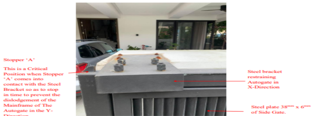
Photo 30 Side Elevation of Steel Bracket
