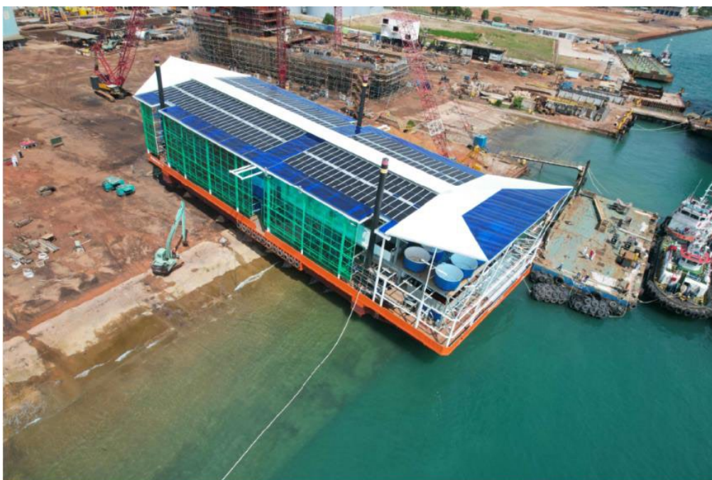
Figure 3B: Photo of the Vessel with three spud legs
