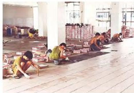
Tile Bonding & Waterproofing at Camel Nut Factory
